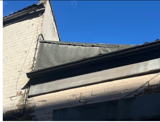
Photo 8 Location: Pitched roof (felt)
