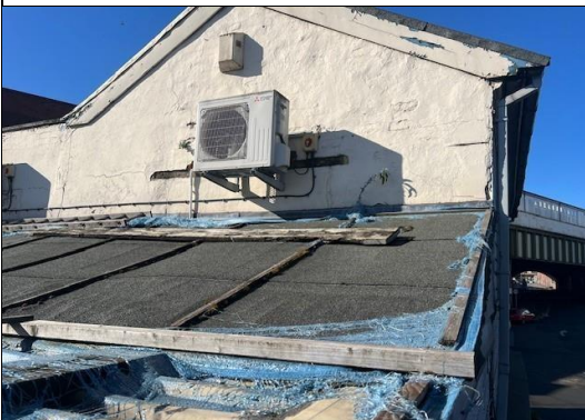
Photo 3 Location: Pitched roof (felt)
