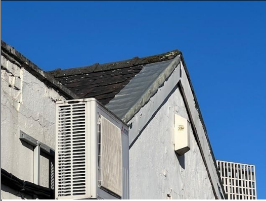
Photo 7 Location: Pitched roof
